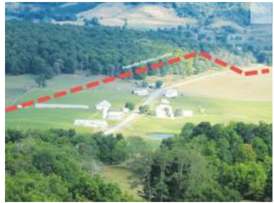
This graphic is one of several now posted to the Highlanders for Responsible Development web site, which was recently updated. It shows the potential pipeline route as proposed by Dominion Resources, where it could cross the historic Dividing Waters Farm in Hightown, owned by the Hevener family.
